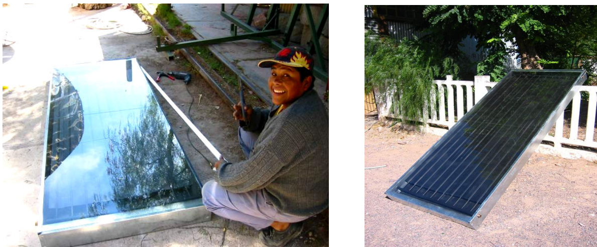
Fig. 6: Hot water collectors built by the co-operative PIRCA/Tilcara
