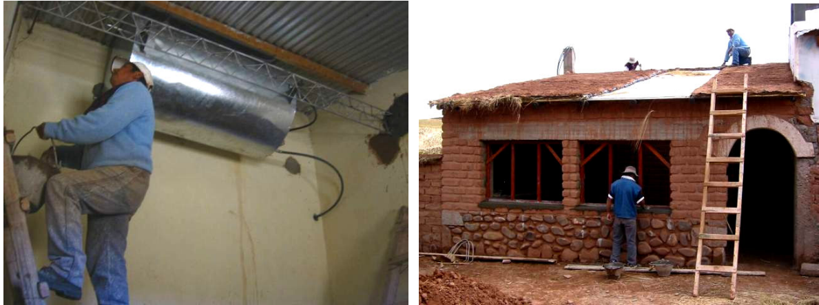
Fig.5. Hot water collector in Cusi Cusi and solar community bathhouse in Cienaga
