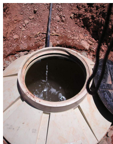
Fig. 11: Solar pump used for irrigation and a 1000 liter tank in Cienaga
